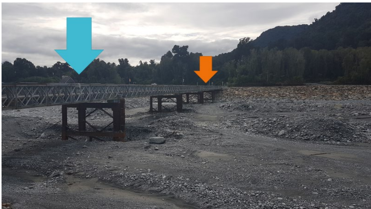
Figure 2: The Waiho River view from the right bank while flow is confined to the left edge of the channel. Sensor locations marked with blue and orange arrows.
